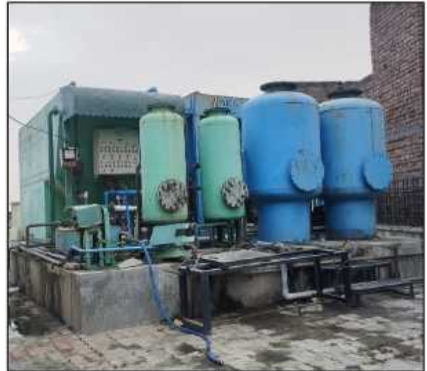
SEWAGE TREATMENT PLANT
